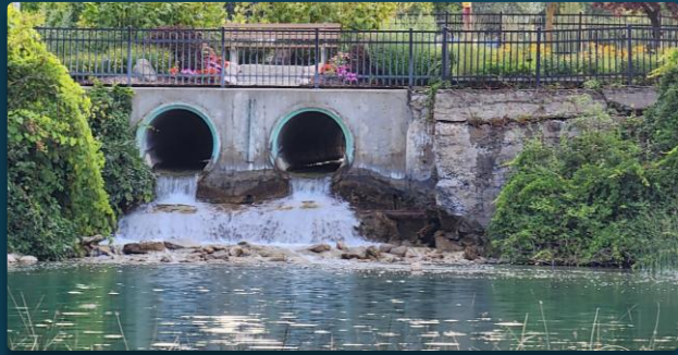
Elk Rapids Overflow Spillway
