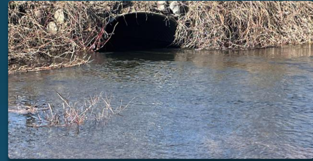
Bridge St. Culvert Ellsworth
